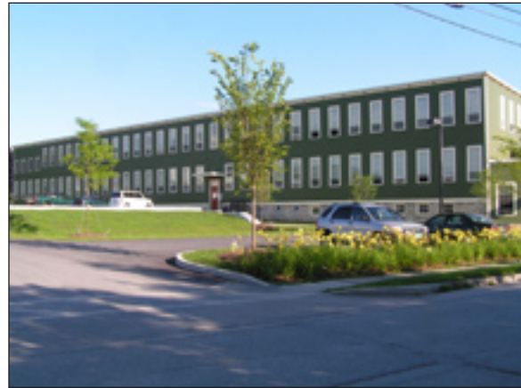
Willard Mill – Innovative and attractive housing complex with 27 apartments near downtown St. Albans; 24 of which are affordable units.
