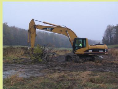
*Fallen trees were placed in and along the stream to trap sediment, provide habitat and help restore the natural condition of the*
