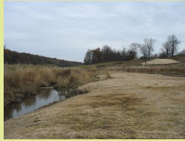
*The berm along the stream was removed to reconnect the stream with its floodplain. Floodplain areas provide space for*
