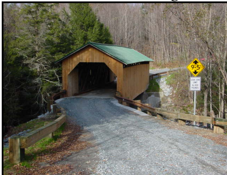
Creamery Bridge Both Restored in 2010
