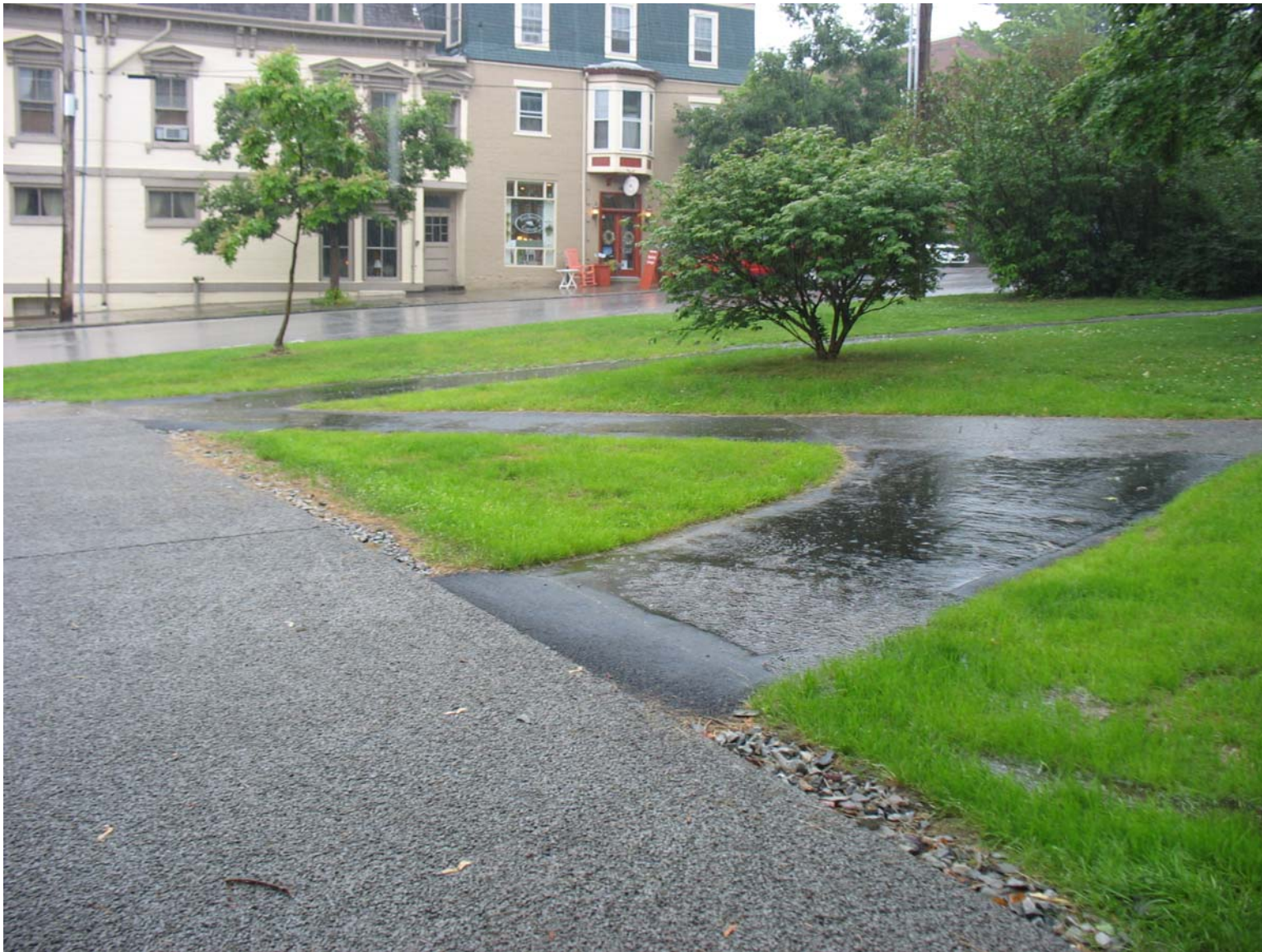
Porous concrete sidewalk in Taylor Park, St. Albans – Notice how wet the asphalt walk is compared to the porous walk.
