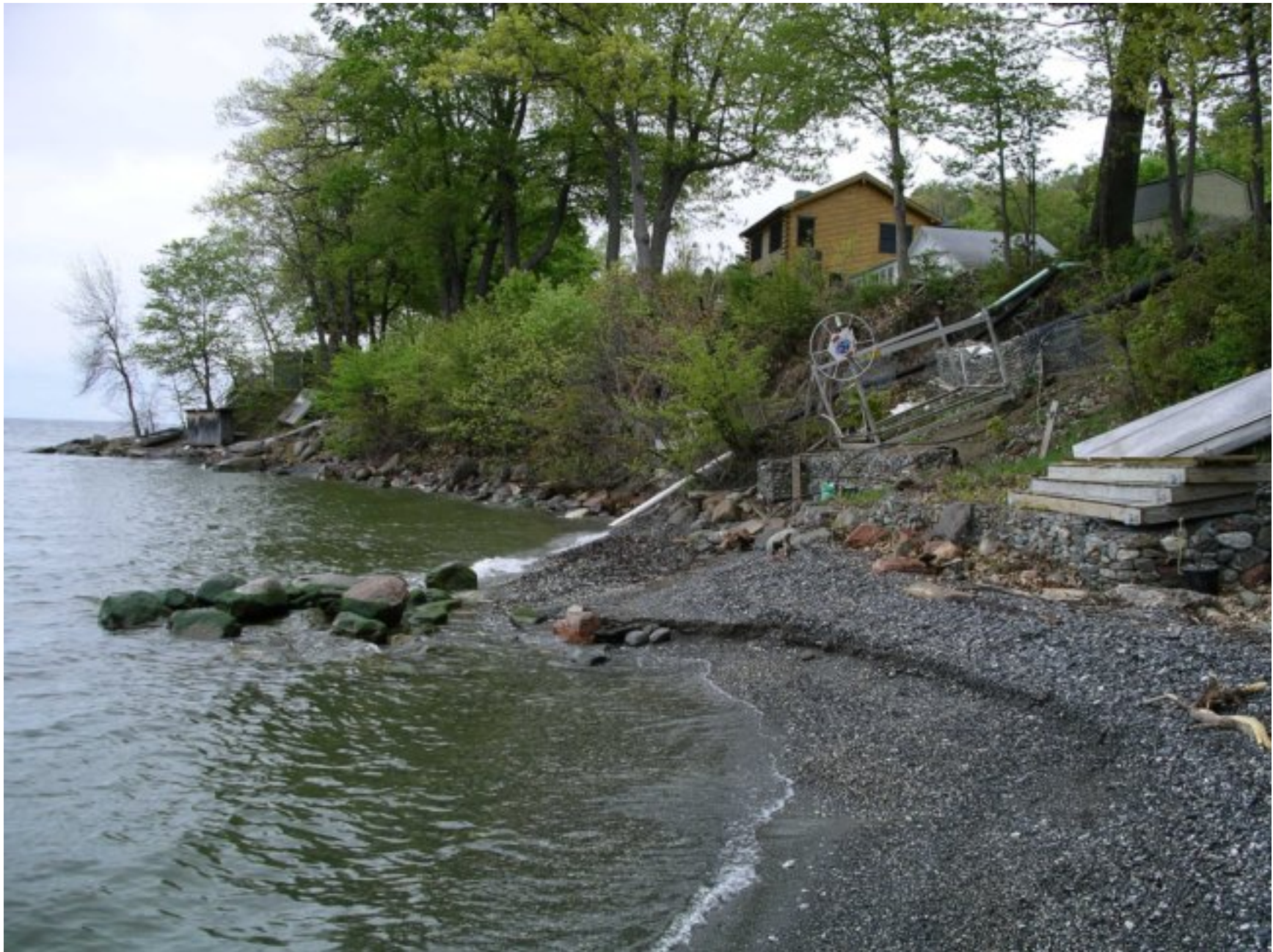
Rock jetty interrupting shoreline drift; notice erosion on this side of jetty
