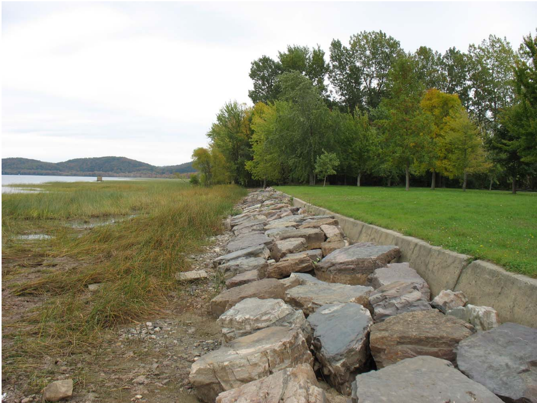
Adapting an existing concrete wall to accommodate ice push
