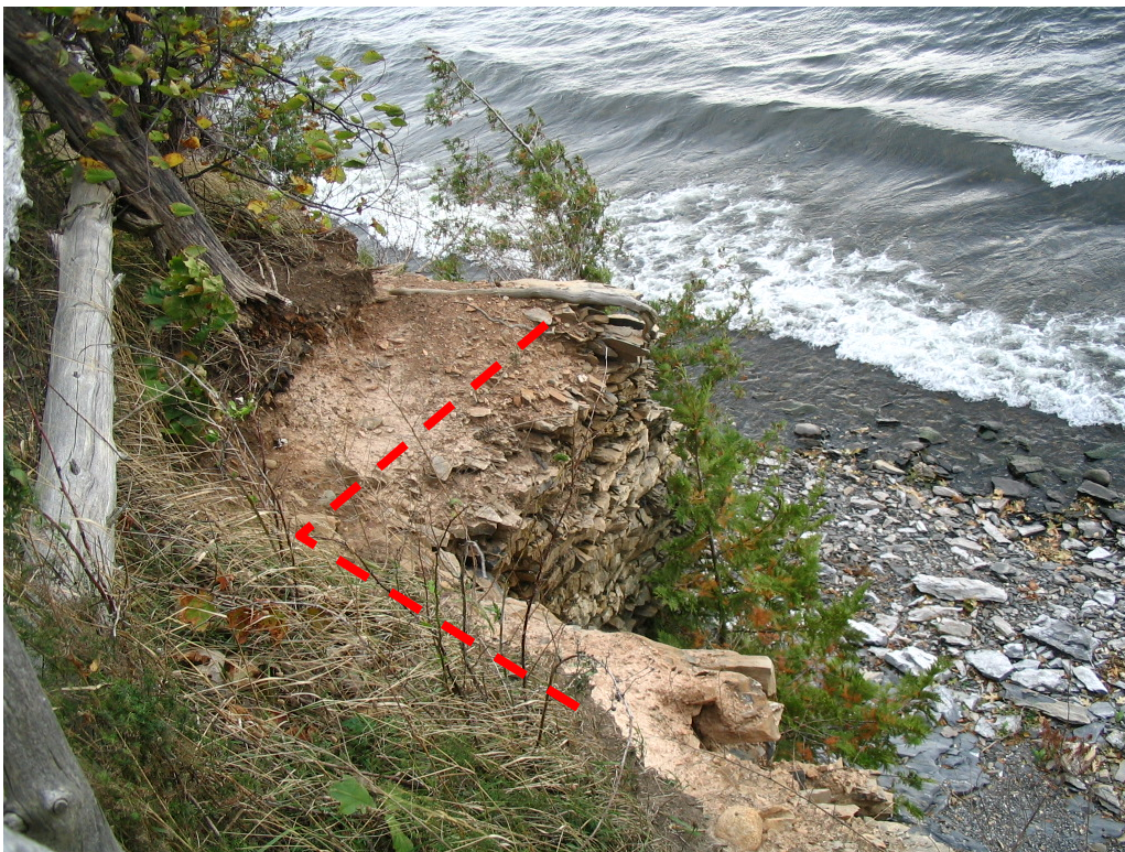
V-shaped notches in the shoreline Indicate a concentration point for water
