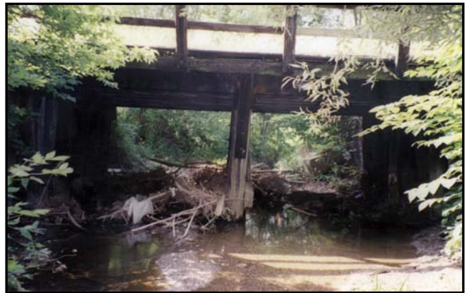
Severely constricted channels and structures trap flood borne debris, causing flooding.
