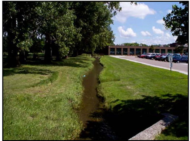
Straightened channels and lack of vegetated buffer reduces ability to filter pollutants from parking lots and contributes to flooding.
