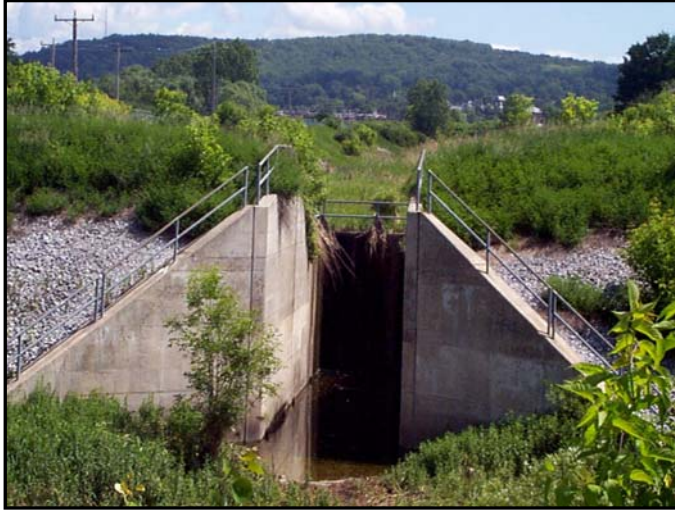
Outlet from the diversion structure.
