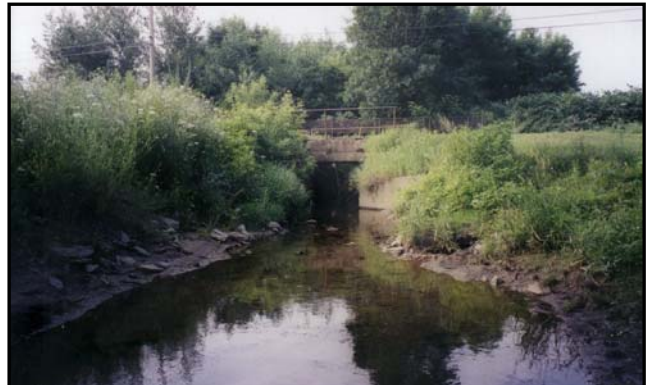
Severely constricted channels and structures trap flood borne debris, causing flooding.
