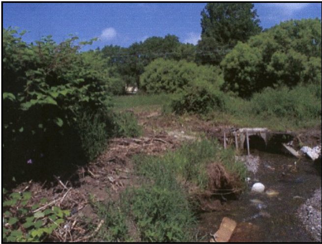
Inlet to diversion structure
