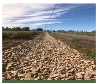
Figure 2.3: This new stone lined ditch on Kibbe Point Road was funded by Grants In Aid in 2022 and will reduce erosion and improve stormwater infiltration.
