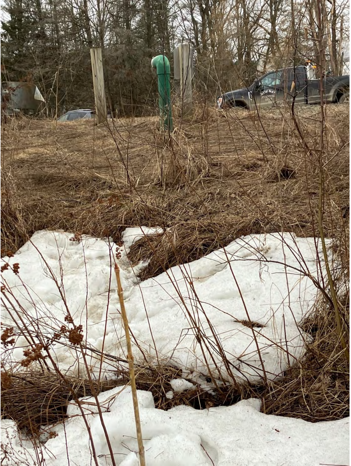
Dry hydrant. Must consider when designing this project.
