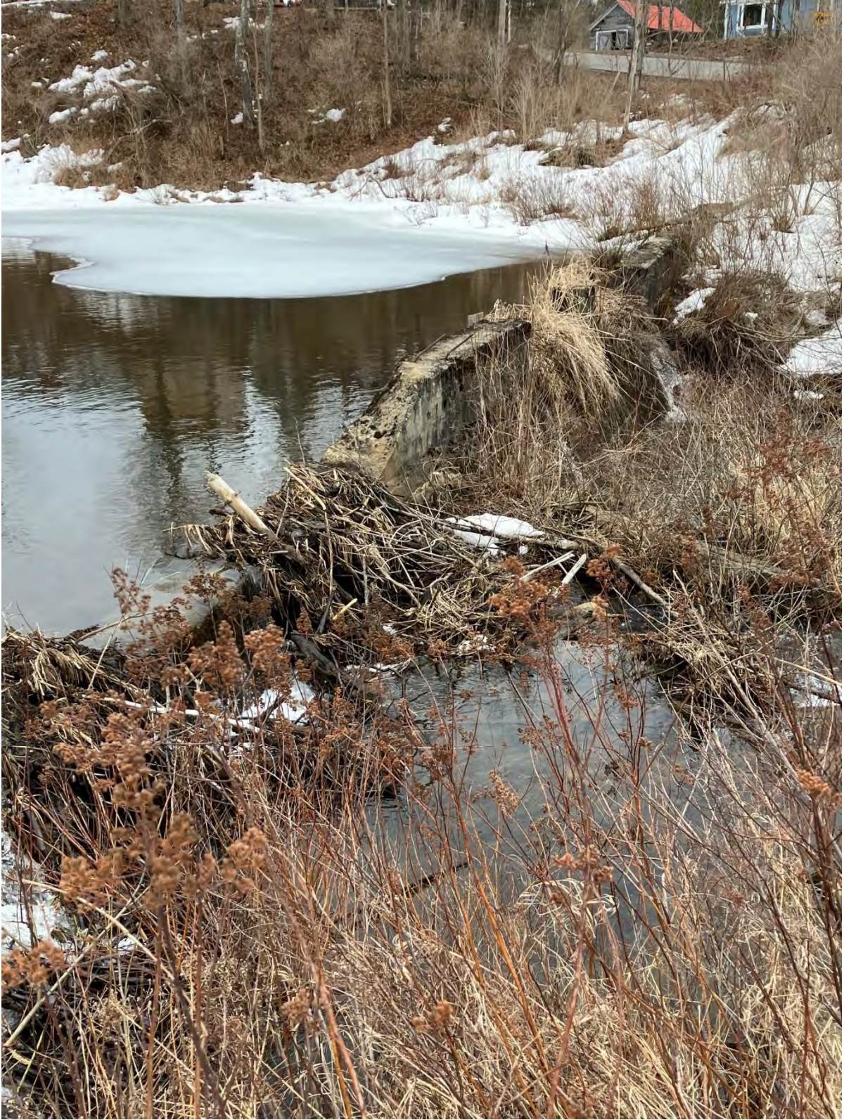
View of the Dam over Centerville Brook
