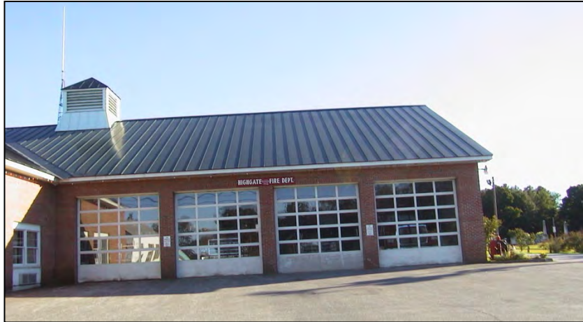
Highgate Fire Department
