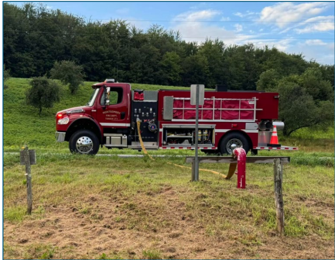
Dry Hydrant, Courtesy Montgomery Fire and First Response
