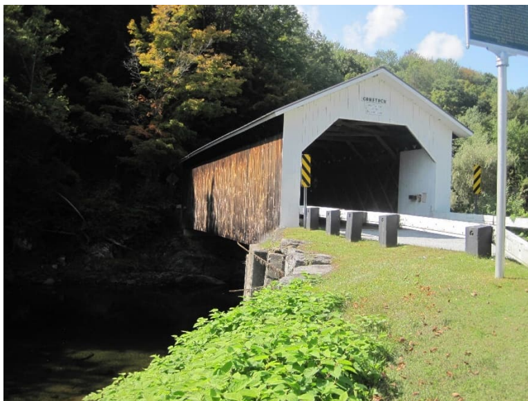
Figure 6. Comstock Covered Bridge.
