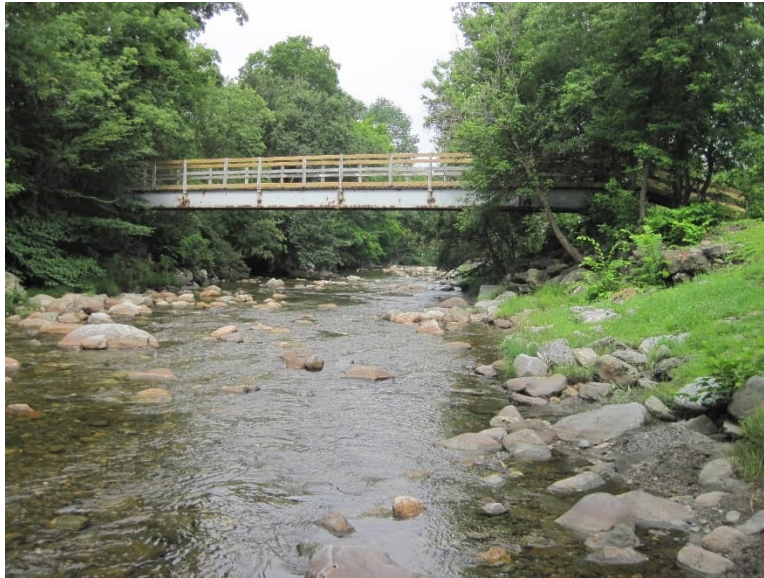
Figure 5. Snowmobile bridge in Montgomery Center.
