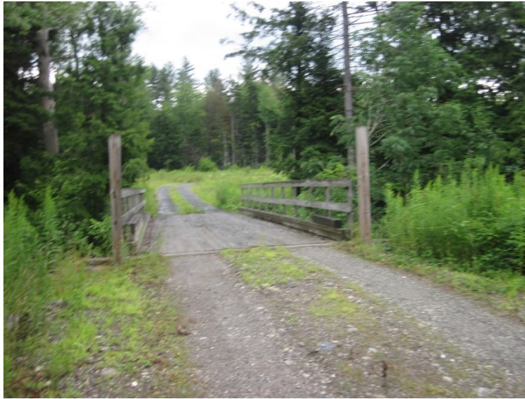
Figure 8. Driveway bridge to 768 Mountain Road.
