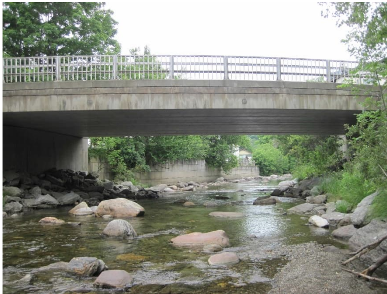
Figure 4. North Main Street Bridge in Montgomery Center.
