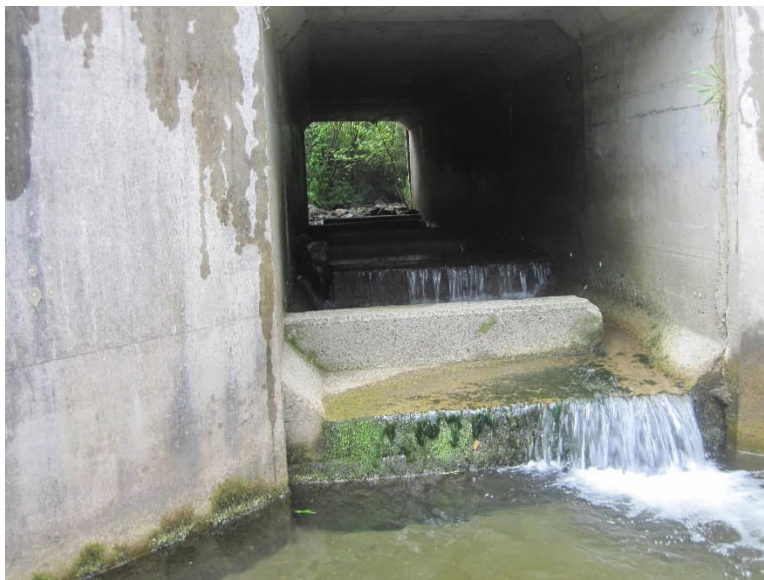
Figure 13. Longley Bridge Road tributary culvert outlet.
