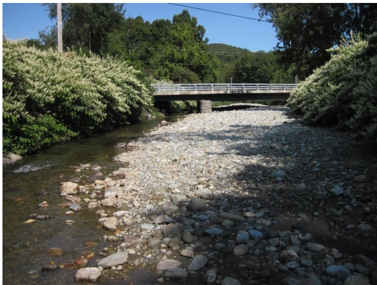
Figure 11. West Hill Brook bridge from upstream.
