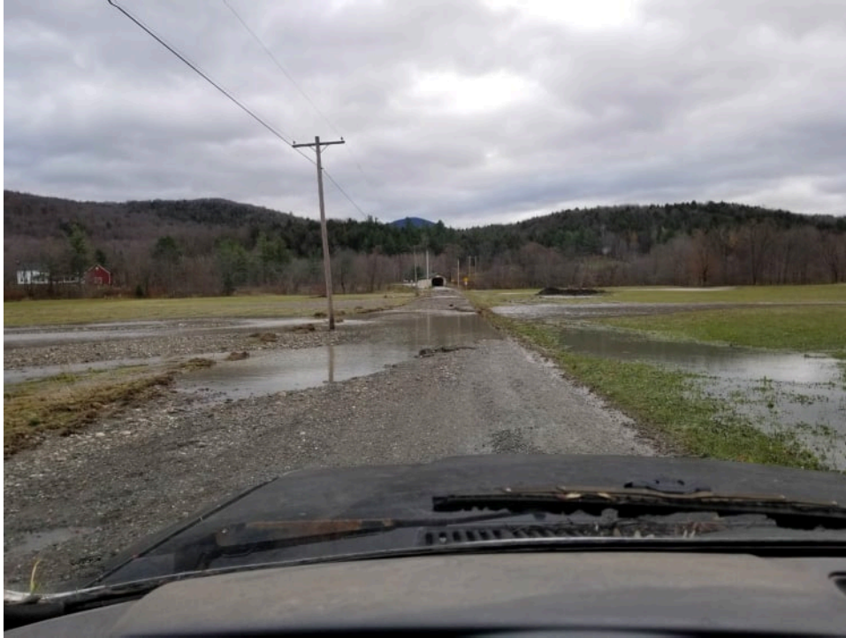
Longley Bridge Road Following Halloween 2019 Flood
