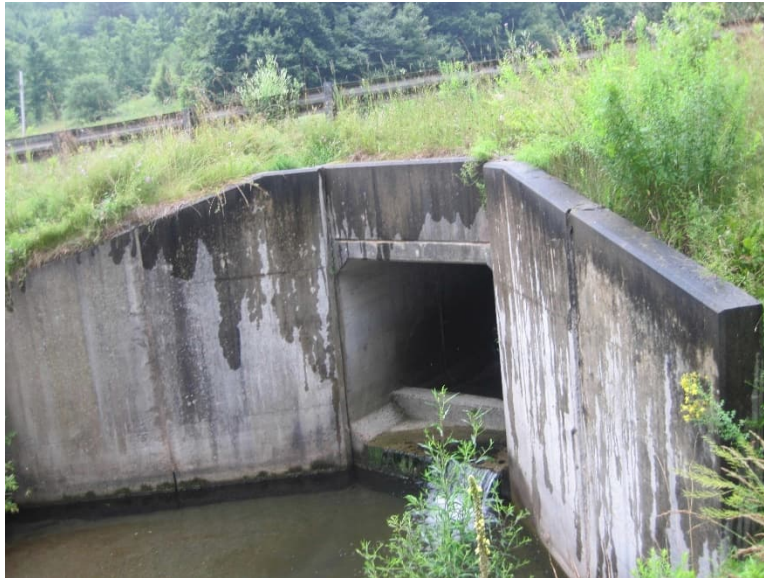
Figure 12. Longley Bridge Road tributary culvert outlet.
