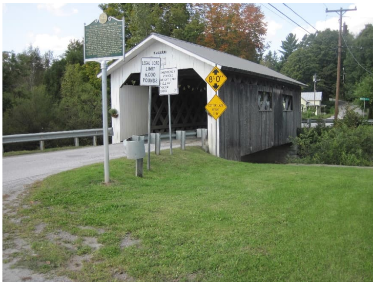
Figure 9. Fuller Covered Bridge.
