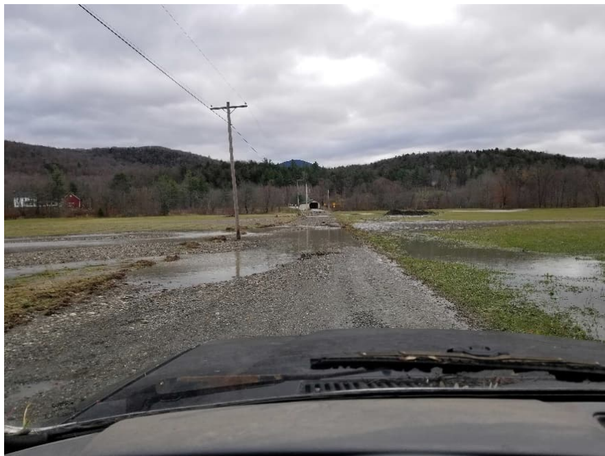
Figure 18. Longley Bridge Road looking east toward the covered bridge at the damaged section of roadway following the Halloween 2019 flood.
