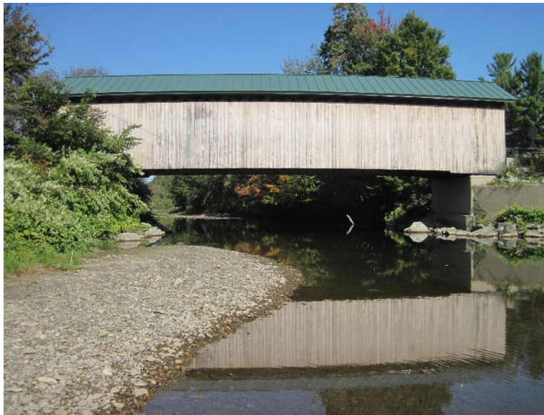
Figure 7. Longley Covered Bridge.
