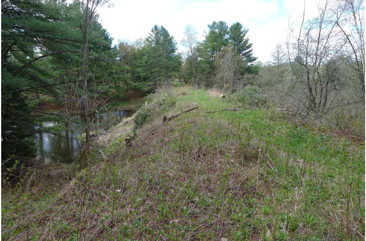
Figure 15. Photo looking south at the existing railroad bed and the southern section of Disposal Area 2, for the proposed Stone J & M Dam Removal Project, North Troy, Orleans County, Vermont.
