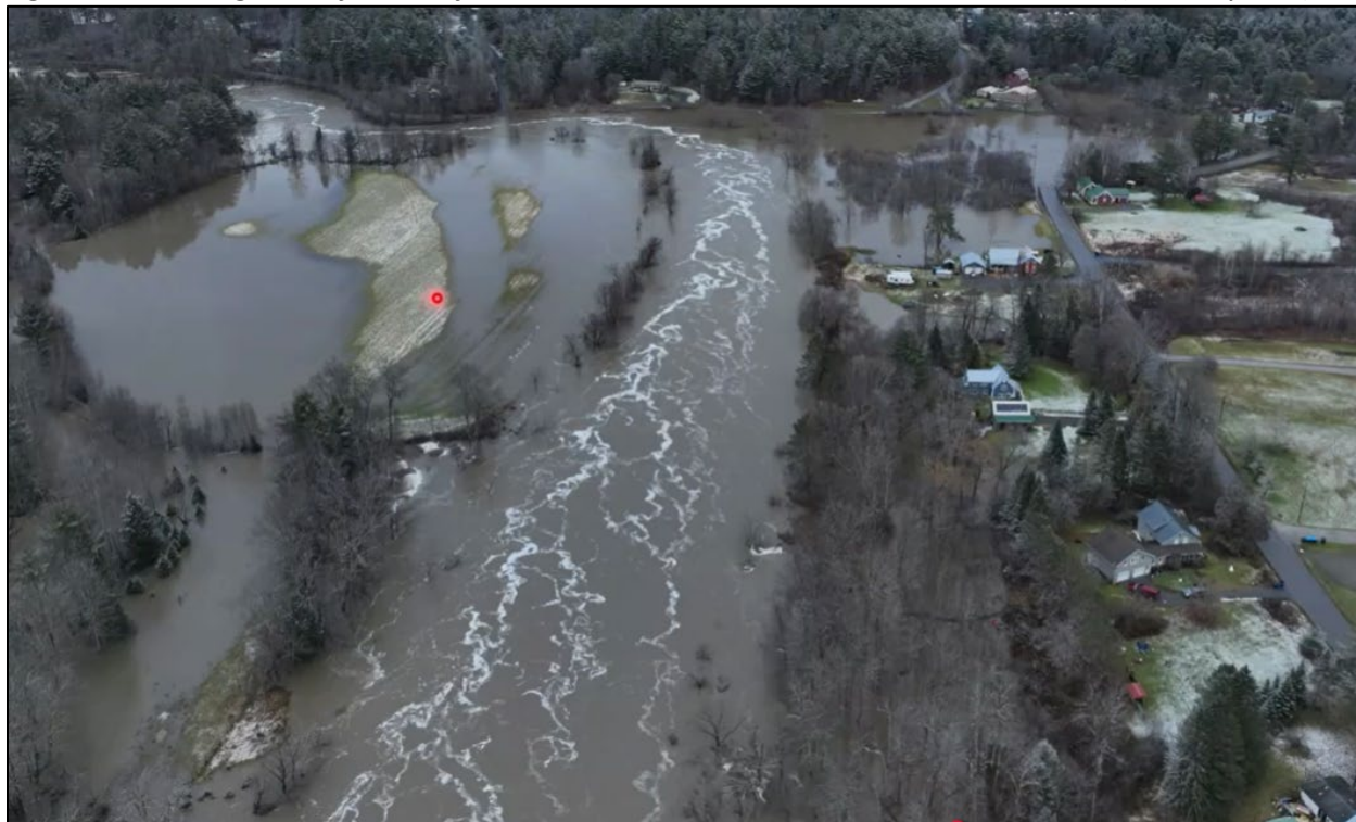
Figure 10: Flooding at Confluence of Stones Brook and Lamoille River, December 2023. (Courtesy: SLR)
