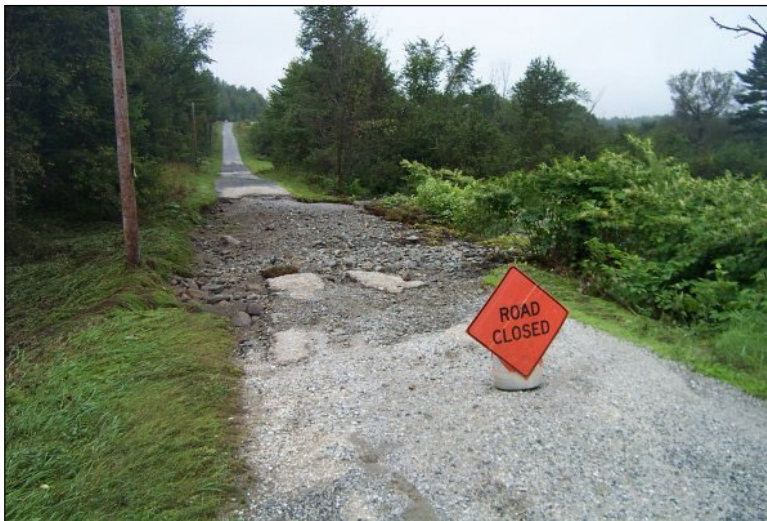
Figure 2: Flooding closes the Fanton Road
