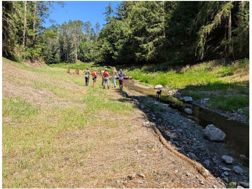
Figure 1 Trout Brook Dam removal
