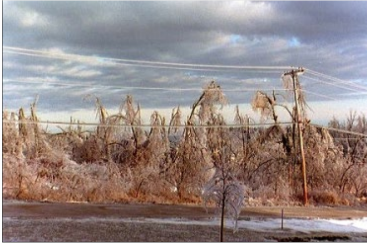
Figure 6: Ice Storm Damage.
