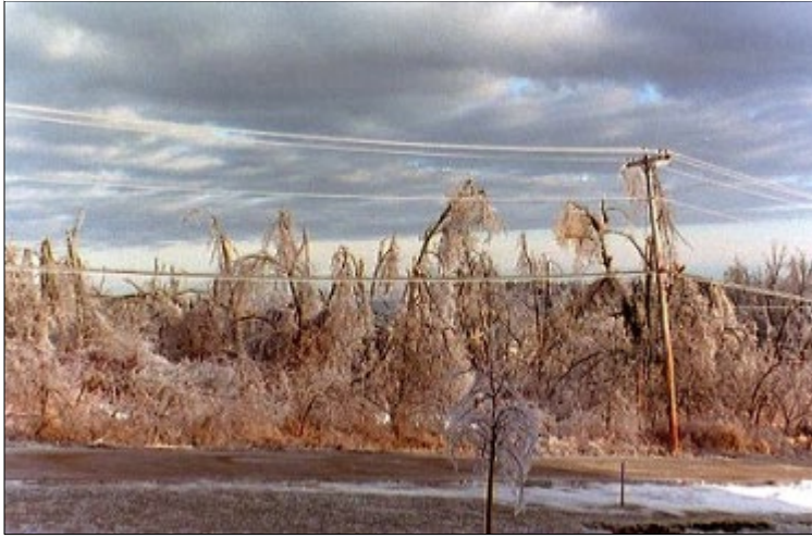
Figure 7: Ice Storm Damage.
